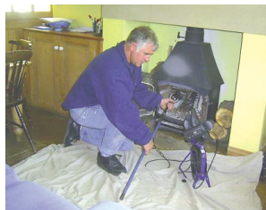
Using CCTV to inspect a chimney for defects.
